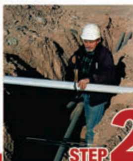
STEP 2 Cut split duct conduit to fit
