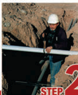
STEP 2 Cut split duct conduit to fit
