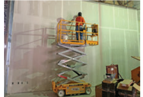
Springfield-based contractor Steel Wall Construction found great success renting the PS-1930 through Superior Rents for a current retail construction job. Photo courtesy of Hy-Brid Lifts.
