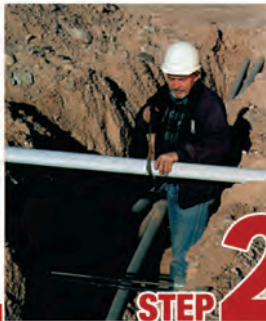
STEP 2 Cut split duct conduit to fit
