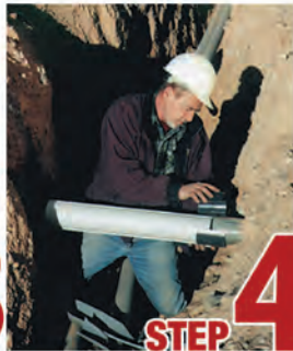
STEP 4 Attach adapters
