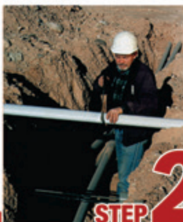
STEP 2 Cut split duct conduit to fit
