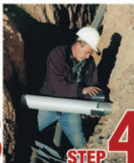
STEP 4 Attach adapters
