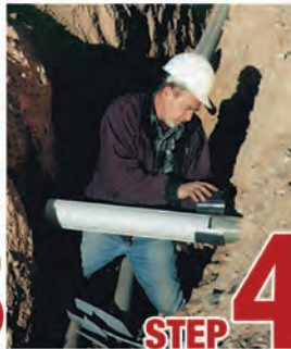
STEP 4 Attach adapters
