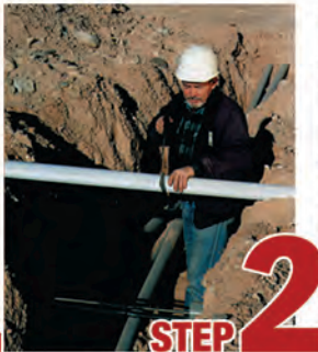
STEP 2 Cut split duct conduit to fit
