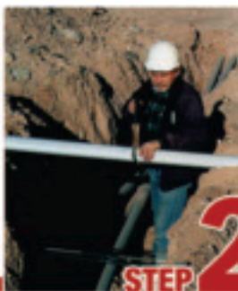
STEP 2 Cut split duct conduit to fit
