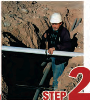
STEP 2 Cut split duct conduit to fit
