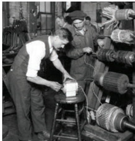
Checking DC motor armatures with a Megger Insulation tester—1930's style!
