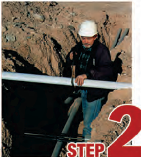
STEP 2 Cut split duct conduit to fit
