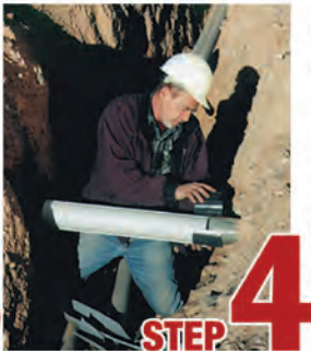
STEP 4 Attach adapters
