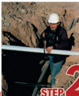
STEP 2 Cut split duct conduit to fit
