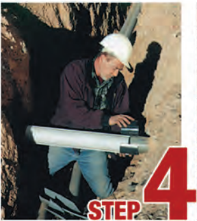
STEP 4 Attach adapters
