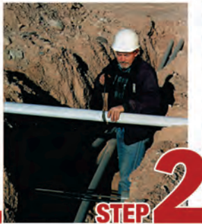
STEP 2 Cut split duct conduit to fit
