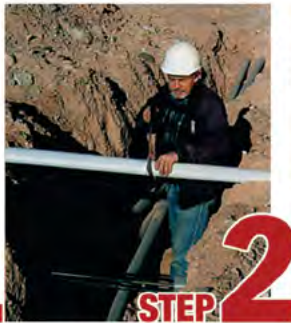
STEP 2 Cut split duct conduit to fit
