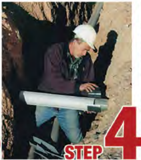
STEP 4 Attach adapters
