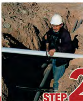
STEP 2 Cut split duct conduit to fit
