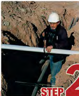
STEP 2 Cut split duct conduit to fit
