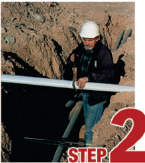
STEP 2 Cut split duct conduit to fit
