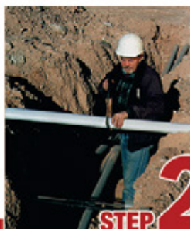
STEP 2 Cut split duct conduit to fit
