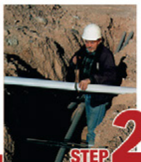
STEP 2 Cut split duct conduit to fit
