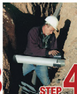
STEP 4 Attach adapters
