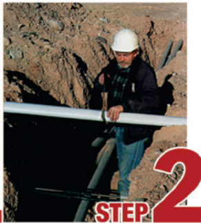
STEP 2 Cut split duct conduit to fit
