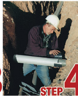
STEP 4 Attach adapters
