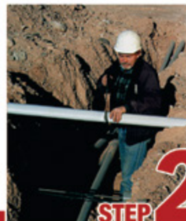
STEP 2 Cut split duct conduit to fit
