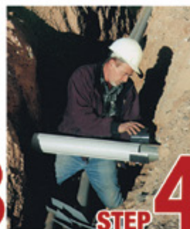
STEP 4 Attach adapters
