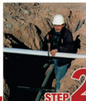
STEP 2 Cut split duct conduit to fit
