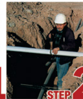
STEP 2 Cut split duct conduit to fit
