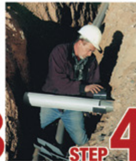
STEP 4 Attach adapters
