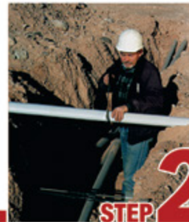
STEP 2 Cut split duct conduit to fit
