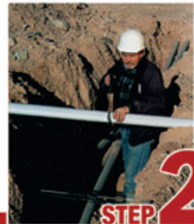
STEP 2 Cut split duct conduit to fit
