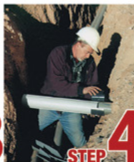
STEP 4 Attach adapters
