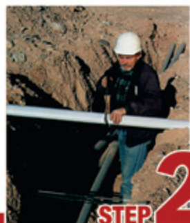
STEP 2 Cut split duct conduit to fit
