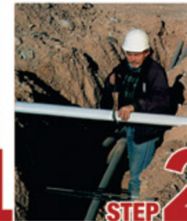
STEP 2 Cut split duct conduit to fit
