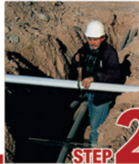
STEP 2 Cut split duct conduit to fit
