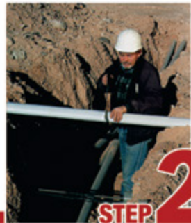
STEP 2 Cut split duct conduit to fit
