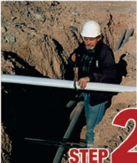
Cut split duct conduit to fit
