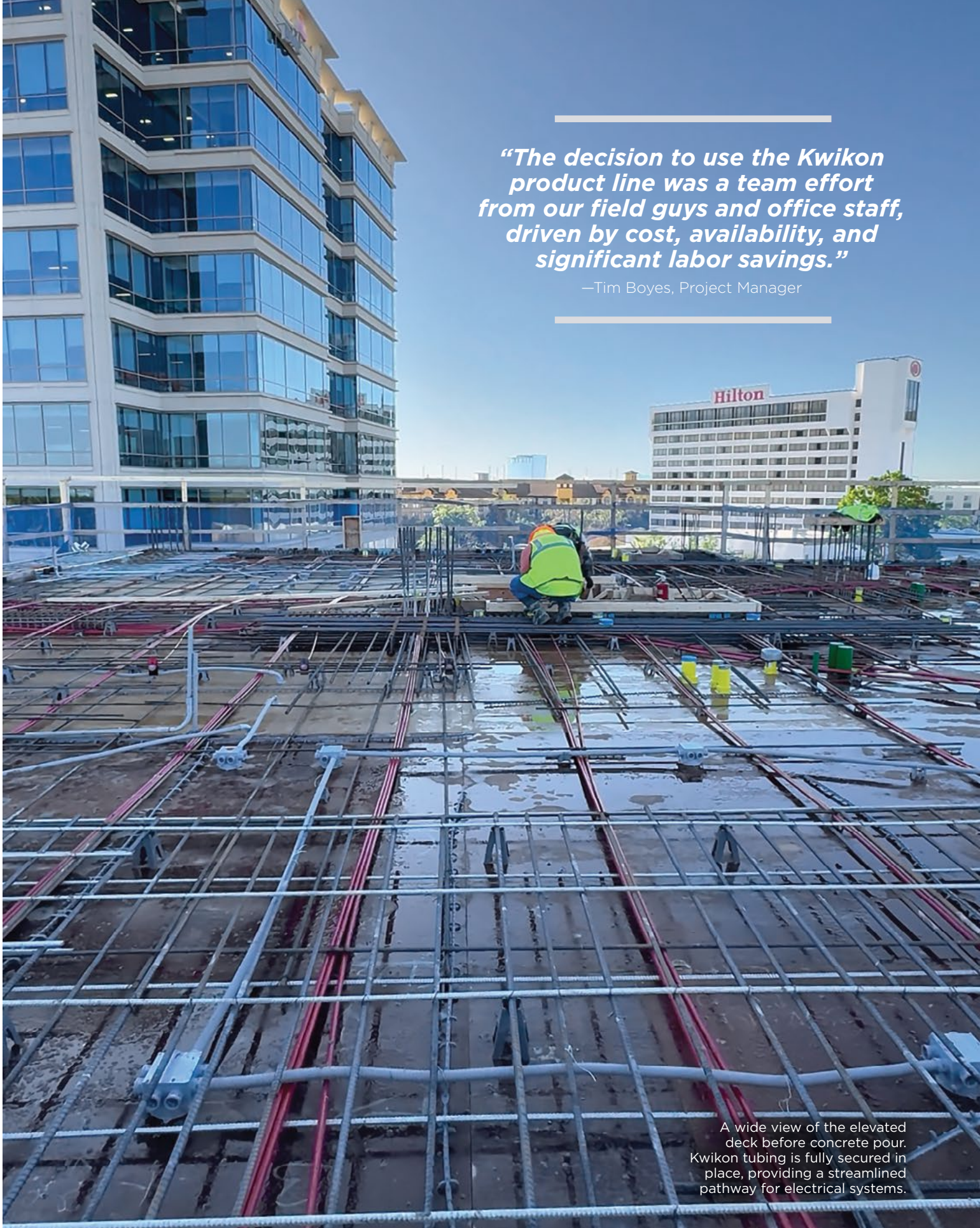
A crew member installs Kwikon ENT between rebar grids. ENT's unique construction allow for fast, tool-free installation.
