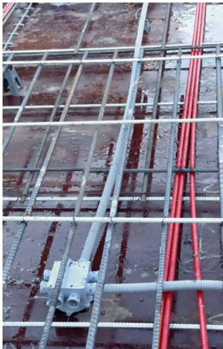
Kwikon ENT connects into electrical slab boxes using snap-in fittings with 6 locking tabs for secure connections perfectly suited for concrete encasement.
