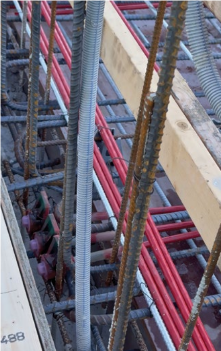
Kwikon ENT fixed to vertically placed rebar.
