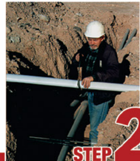
Cut split duct conduit to fit
