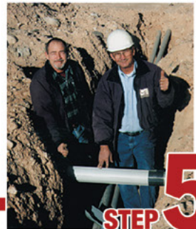
Finish job in record time
