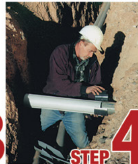
STEP 4 Attach adapters
