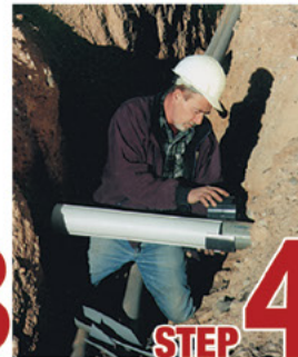
STEP 4 Attach adapters
