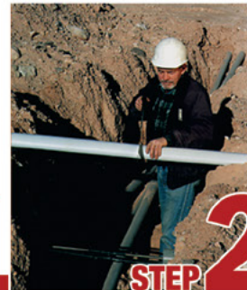
STEP 2 Cut split duct conduit to fit
